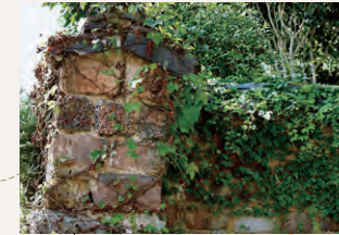
Tonbaibe Wall: in the past when a kiln was dismantled at the end of its working life, bricks from the kiln structure were reused to build walls – an intelligent use of materials unique to pottery areas
