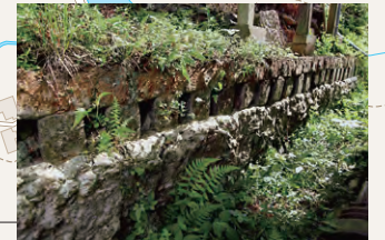
Mikawachi East Kiln Site: the largest multi-chambered climbing kiln stretching to 120m in length, used from the Edo to Shōwa periods (until the mid 20th century). The smoke outlets remain in one section
